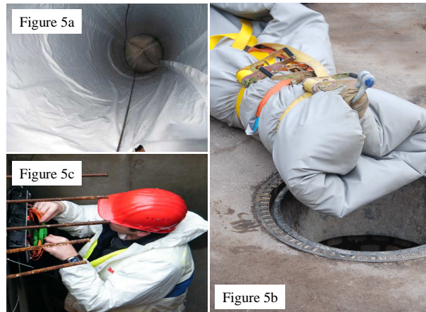
Figure 5: Feeding the sensor cable into the sewage channel.
